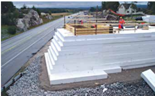
Grimsoyveien Köprüsü (Kaynak: Damtew, T., Vaslestad, J. & Refsdal, G., 2011. Case histories with EPS geofoam embankments from eastern Norway. Proceedings of the 4th International Conference on Geofoam Blocks in Construction Applications, Lilleström, Norway).
